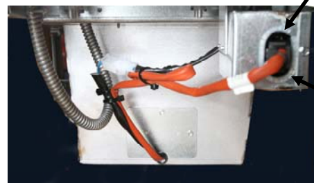
Figure 3: Plug the black connector into the utility box as shown. A separate harness with a white plug, if present, is NOT used.
